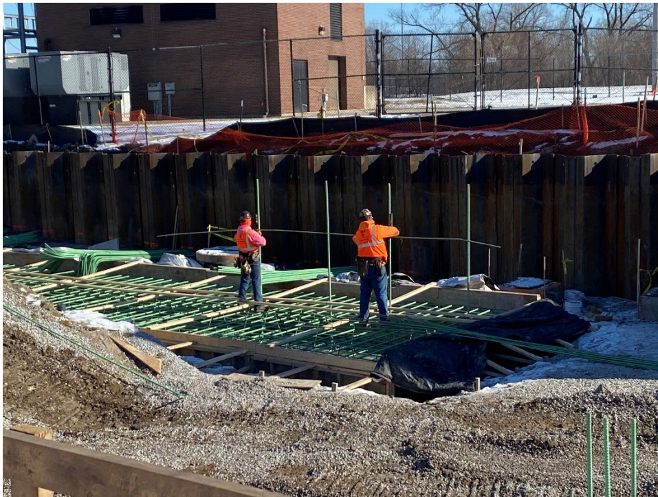
Workers installing rebar for the retaining wall for the ramp on the north side of the tunnel.
