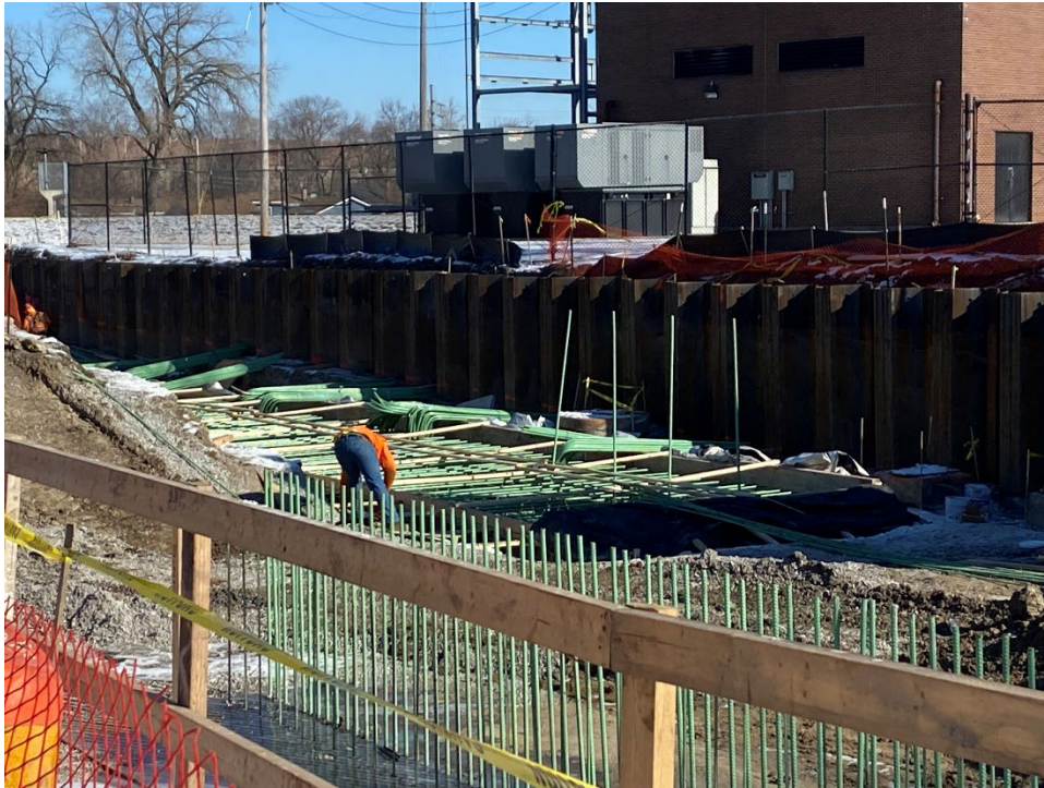
Workers installing rebar for the retaining wall for the ramp on the north side of the tunnel.
