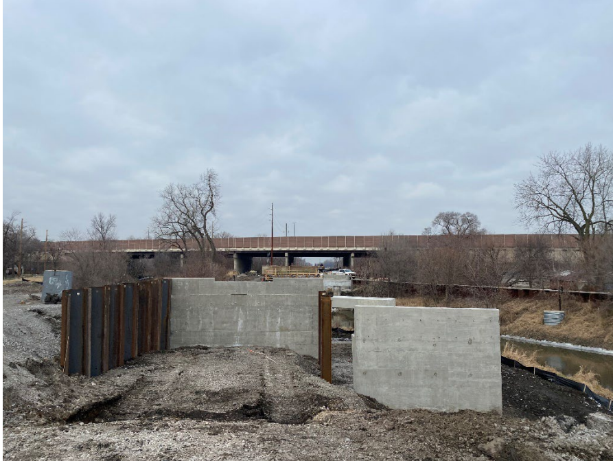
Bridge piers on south side of Little Calumet River. Pier on the left, with the sheeting, is for the train bridge. Pier on the right is for the pedestrian bridge.
