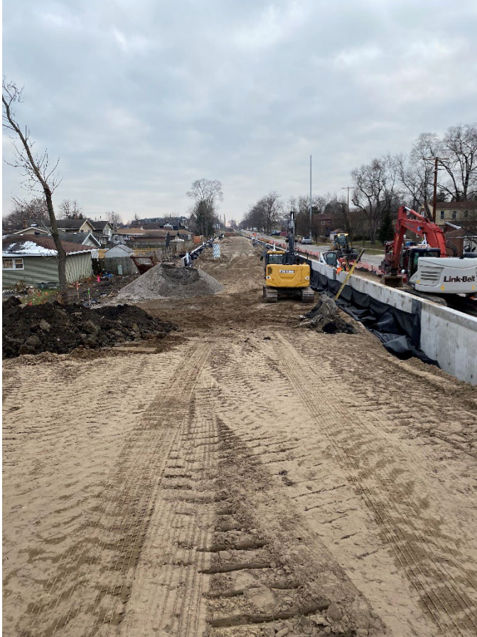
Backfilling behind retaining walls. Belden tunnel looking south.
