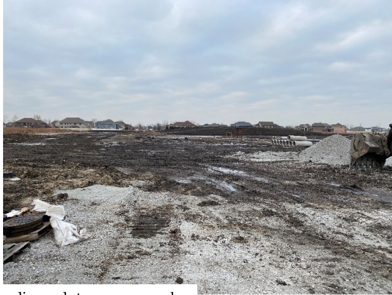
Rough grading and storm sewer work at Main Street station parking lot.
