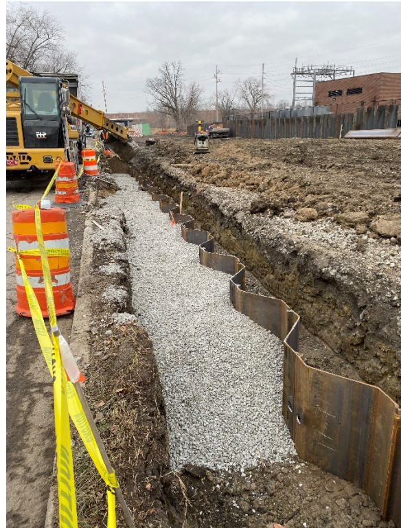
Sheeting for retaining walls at new pedestrian tunnel (between Sunnyside and Fairbanks)
