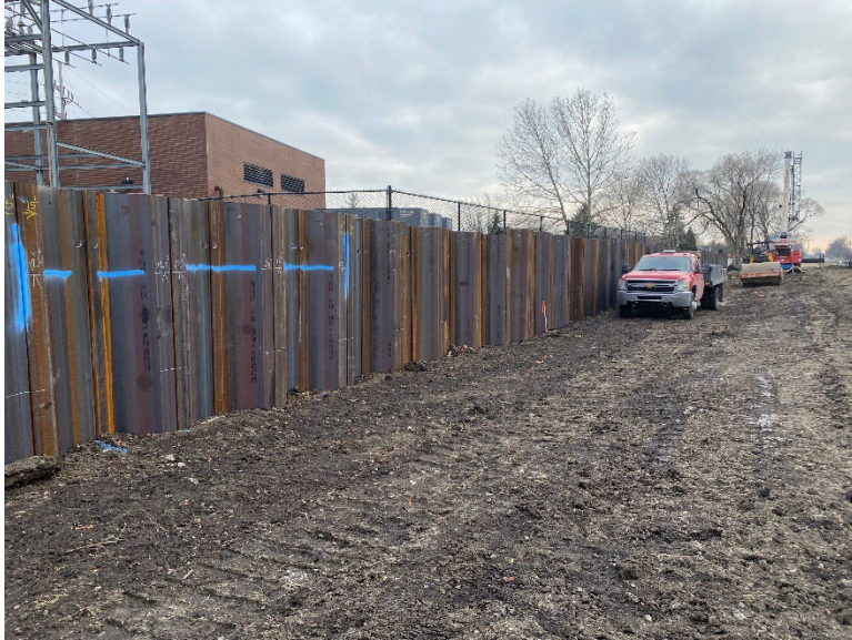
Sheeting for retaining walls at new pedestrian tunnel (between Sunnyside and Fairbanks)
