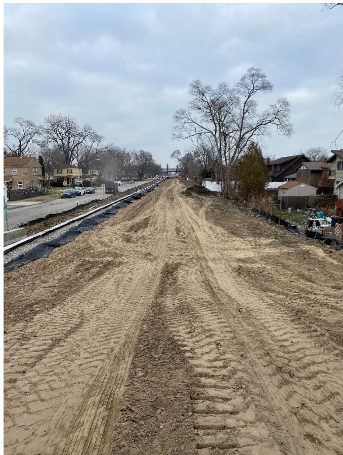
Backfilling behind retaining walls. Belden tunnel looking north.
