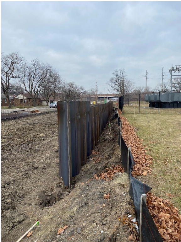
Sheeting for retaining walls at new pedestrian tunnel (between Sunnyside and Fairbanks)
