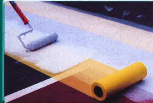
STEP 7: Install yellow ARMOR ® mesh
