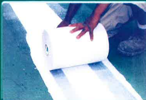
STEP 5: Install narrow ARMOR ® fabric
