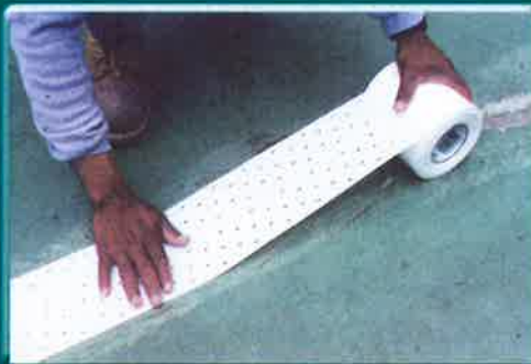
STEP 3: Apply ARMOR ® release tape
