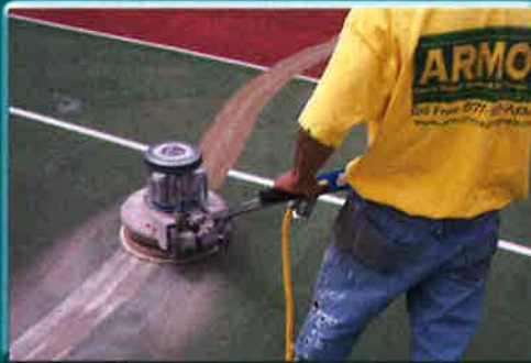
STEP 2: Sand flush to surface
