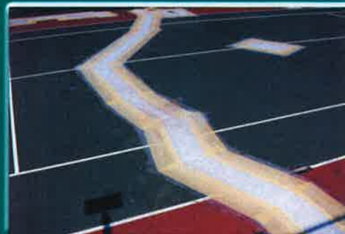
STEP 8: Finished...ready to color coat!
