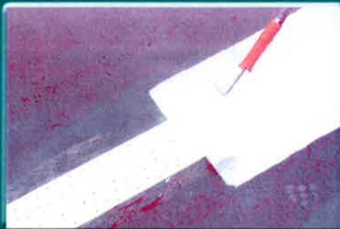
STEP 4: Apply liquid adhesive
