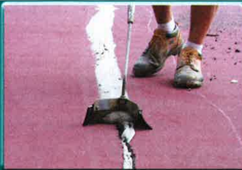
STEP 1: Fill cracks up to 4 inches wide
