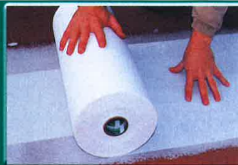
STEP 6: Install wide ARMOR ® fabric
