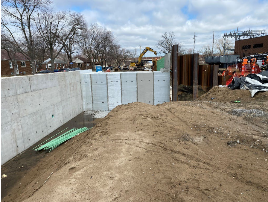
Side view of tunnel. This area will be backfilled with sand and the tracks will be installed over the tunnel.
