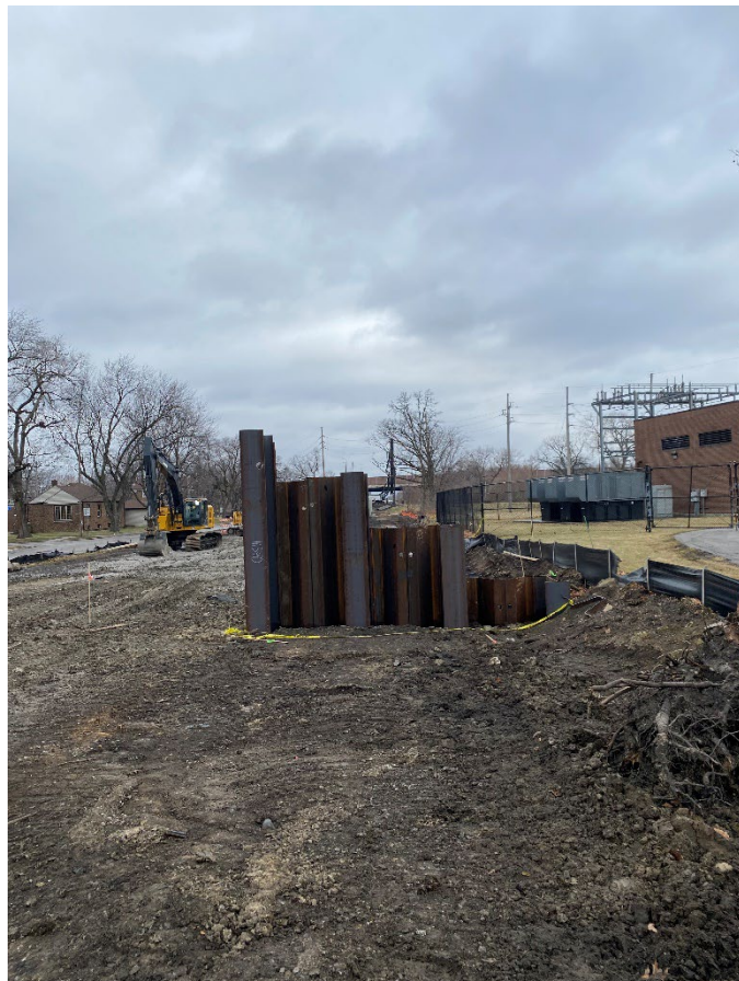
Sheet piles for new pedestrian tunnel at Sunnyside/Fairbanks. Tunnel will be installed to the left.
