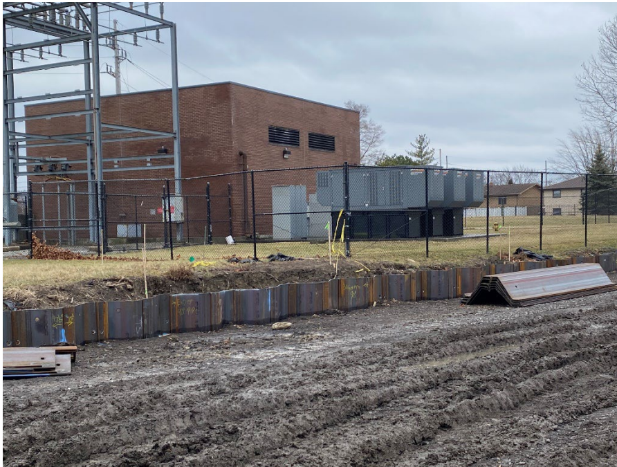
Sheet piles/retaining wall for Monon Trail.
