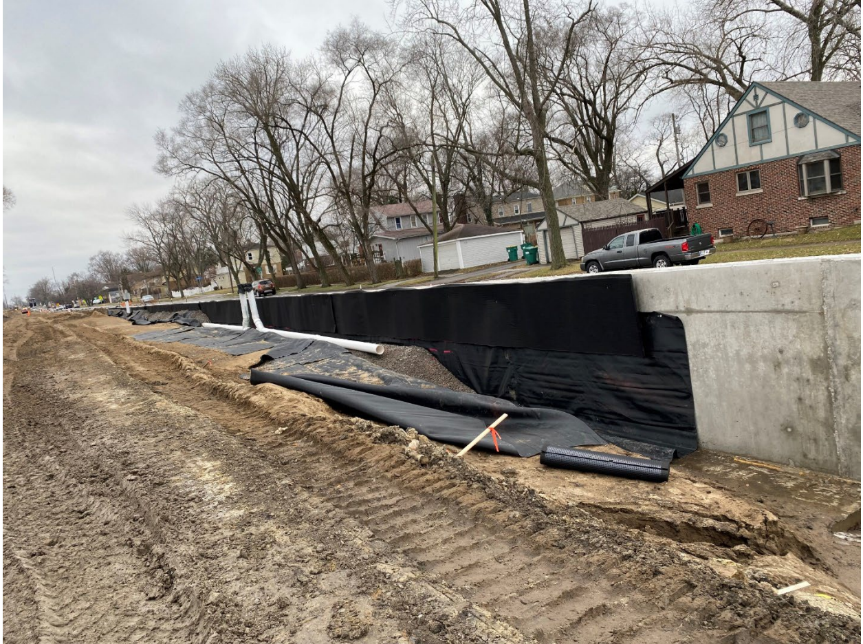
Backfill/drainage behind Manor Avenue retaining wall.
