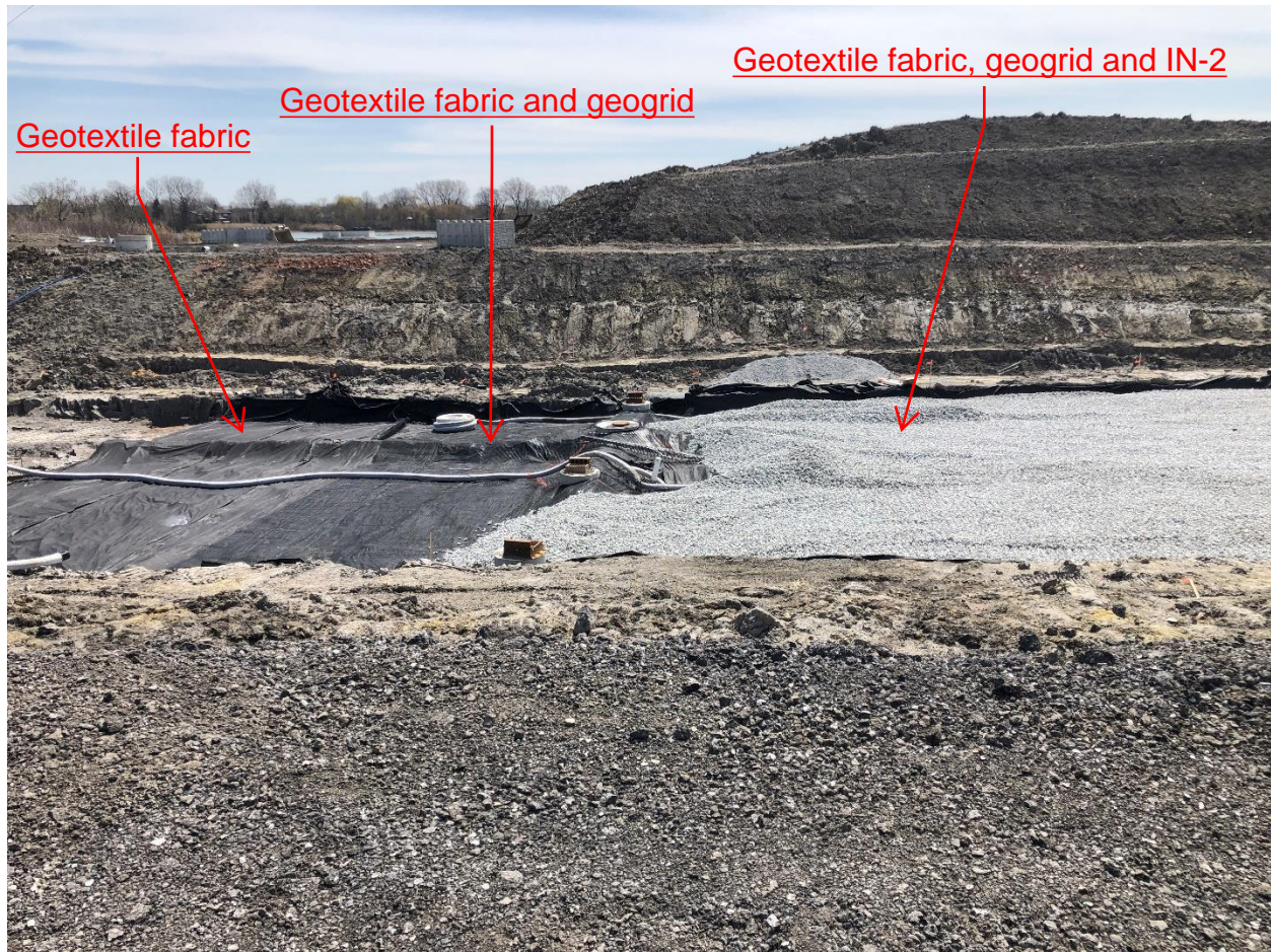
30" undercut of existing soils replaced with geotextile fabric, geogrid and IN-2 between proposed underpass and Centennial Village.
