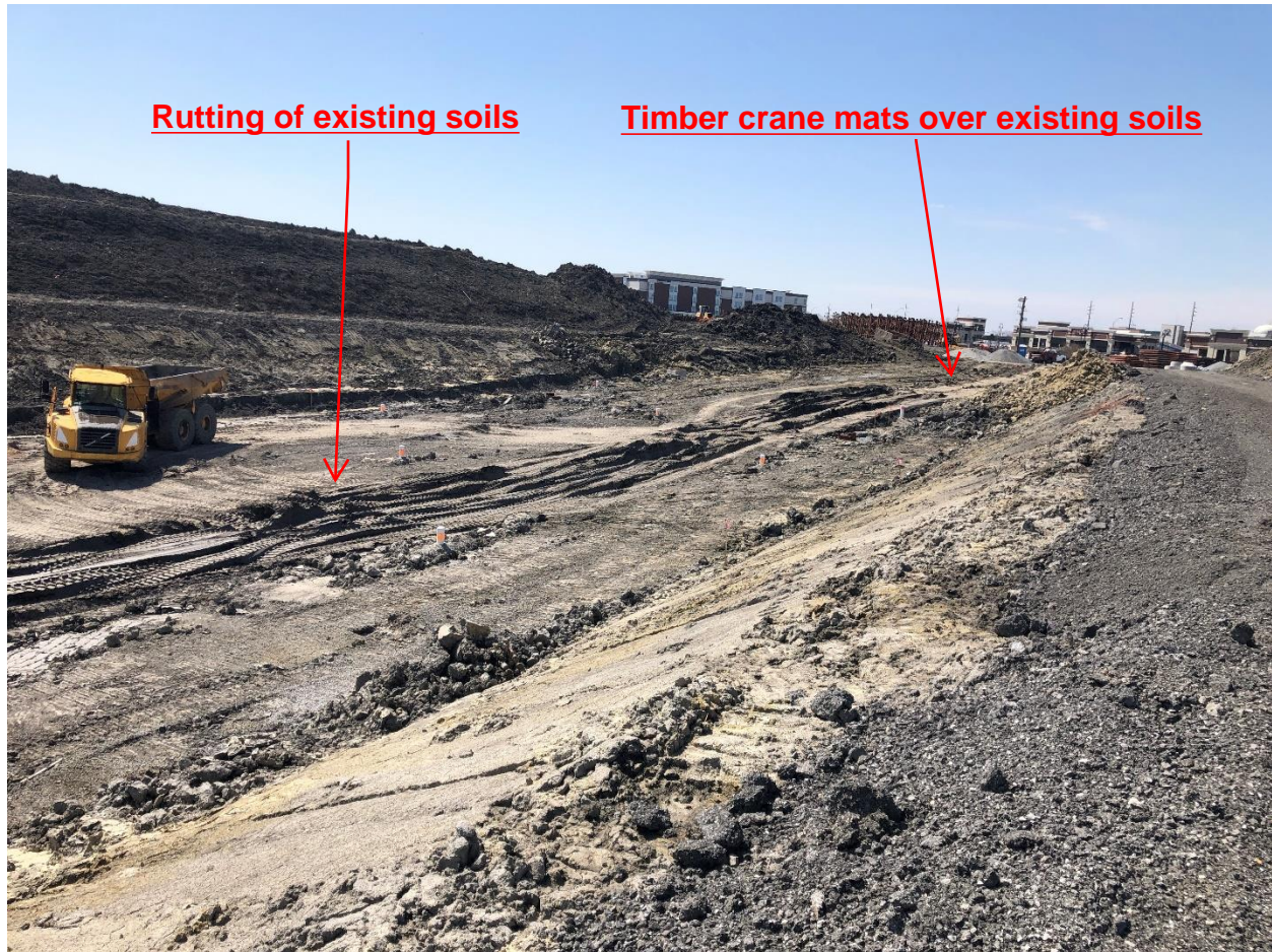
Existing soil conditions rutting under construction traffic – proposed 45 th St between underpass and Centennial Village.
