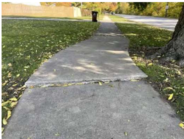
Adjacent sidewalks along Grove Park are heaving and uneven
