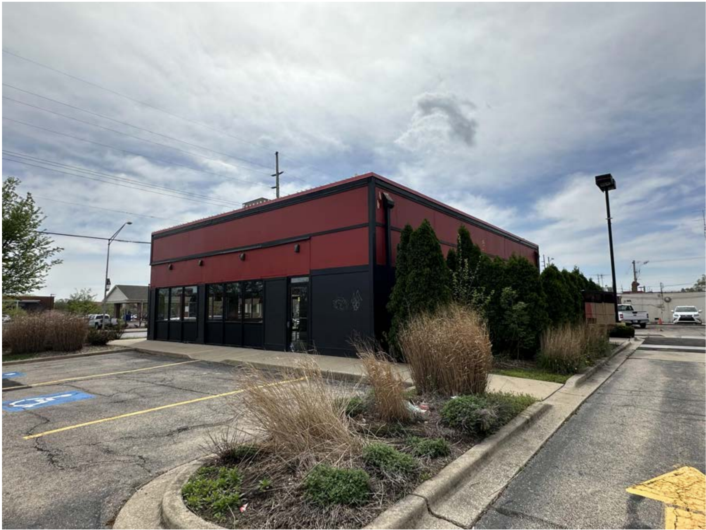
2 EXISTING PHOTO NE VIEW NTS
