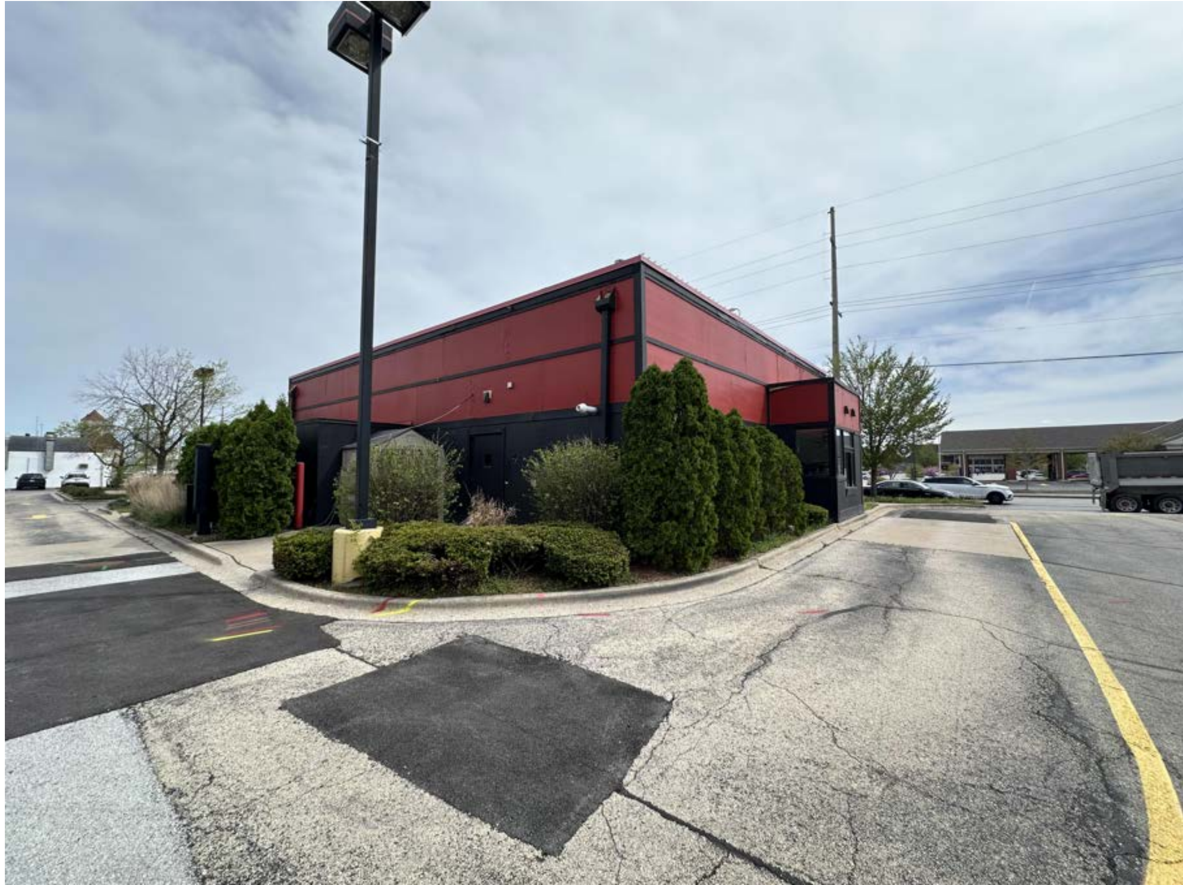
1 EXISTING PHOTO NW VIEW NTS
