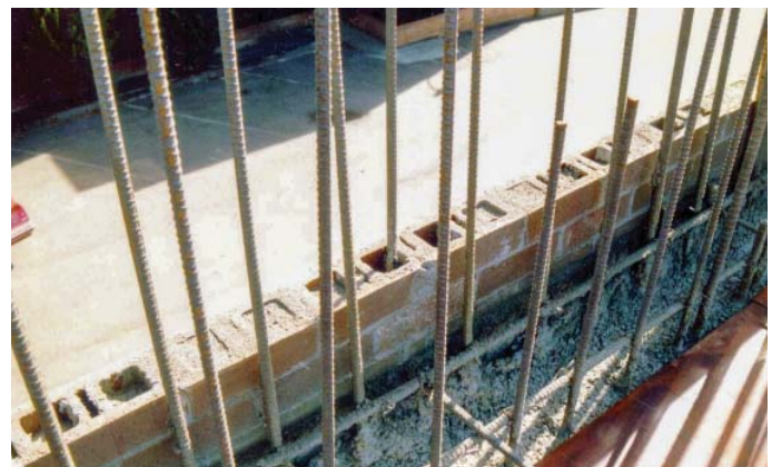
Figure 21 RHCM Used as the Finish Wall and Backing for Concrete Shotcrete (Guniting)
