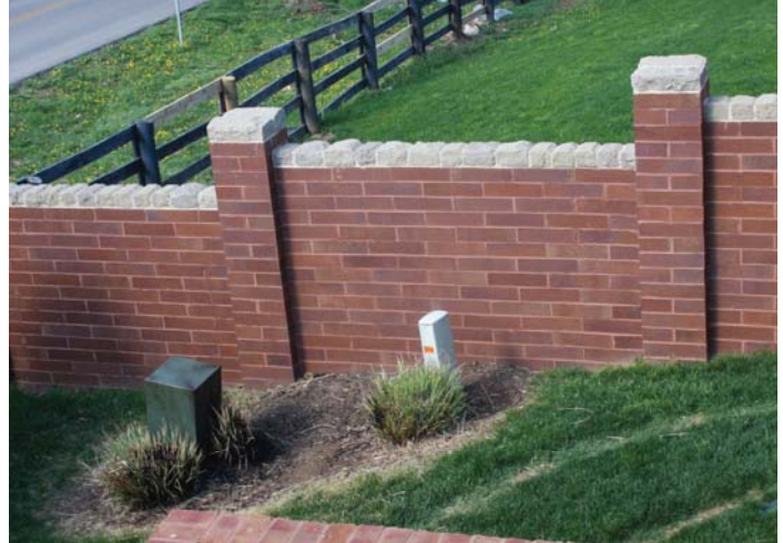
Figure 10 Pier and Panel Sound Wall
