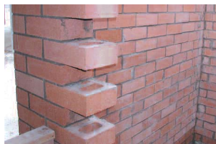
Metro Loft, Royal Oak, constructed of Mission (yellowish, buffish) and Sunset, flashed to bring out color variation. Larger core holes for re-rod and grouting.
