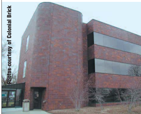
Fox Studio, Livonia, designed by Giffels, Hoyem, Basso, now IDS, Troy, used both 4 x 8 x 16 custom color Brownstone flashed (with center score) as a veneer and 8 x 8 x 16 (with center score) as a structural unit.
