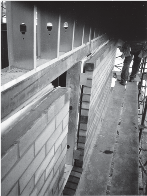
Figure 19 Drift Joint Before Ledger Installation
