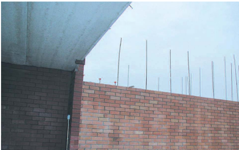
Metro Loft, Royal Oak, designed by Neumann/Smith & Associates. Re-rod and concrete pre-fab flooring attached to 8 x 4 x 12 brick single wythe walls.
