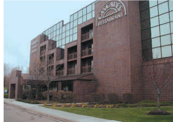
Embassy Suites Hotel, Livonia used both 4" x 8" x 16" Ironstone flashed (with center score) as a veneer and 8" x 8" x 16" (with center score) as a structural unit.
