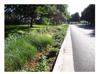
The cross section of the new road will include traditional sidewalk and curb along the outside limits of the pavement, with a natural edge draining to bioswales in the median. We also plan to reconfigure the curb at the intersection with Forest Avenue to reduce the surface area of this intersection and shorten pedestrian pathways through the intersection.
