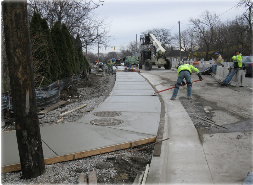
Curb and Gutter with Sidewalk
