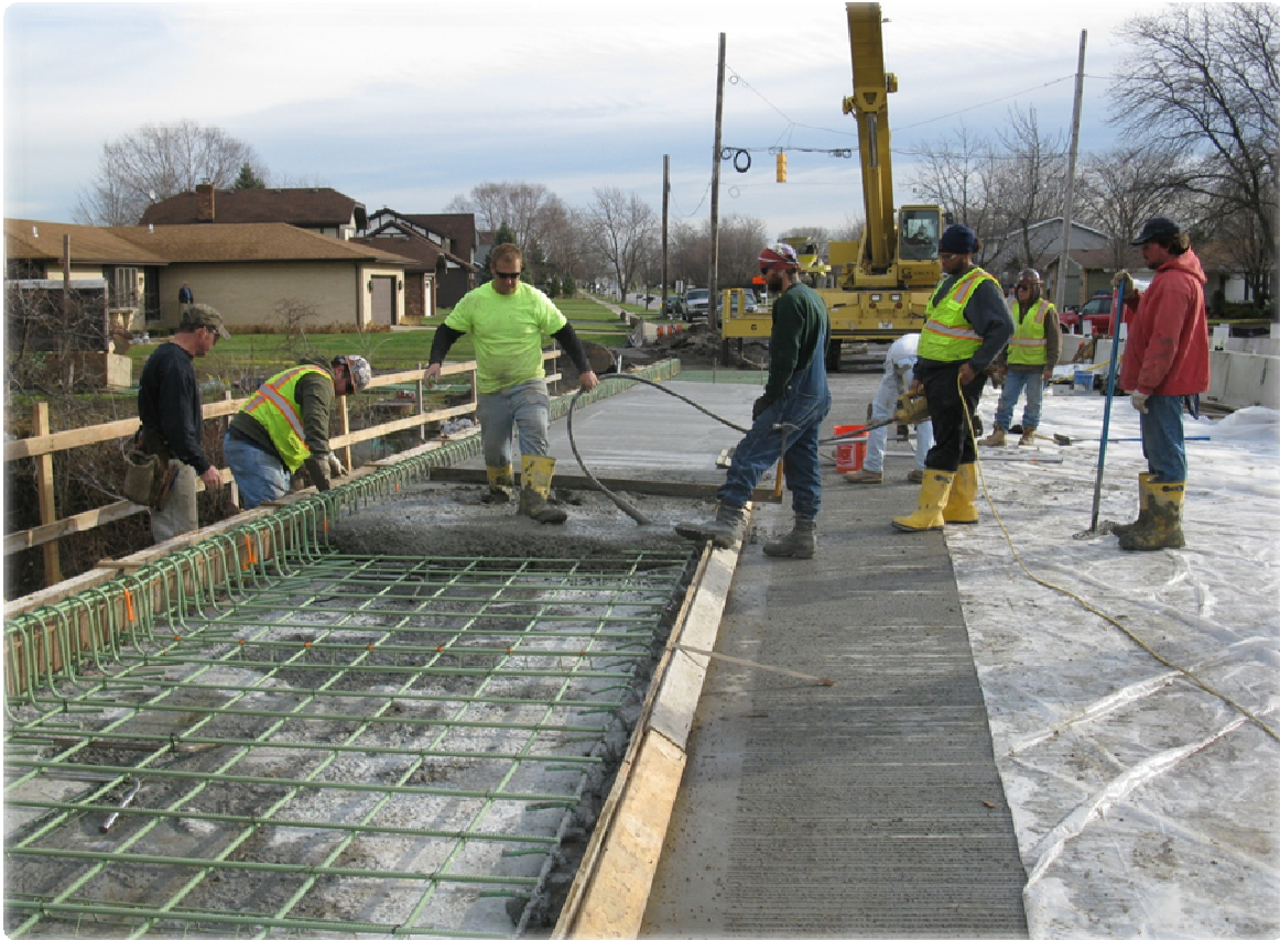
Sidewalk on Bridge and Approaches
